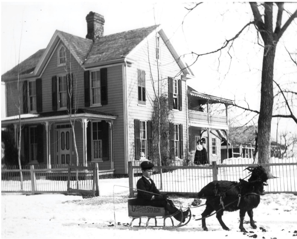
The John S. Hambleton House, built about 1870, had lowered shutters that were hinged and properly sized to cover the window opening.
