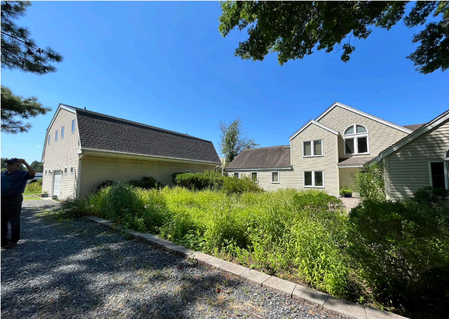
EXISTING SITE IMAGE
