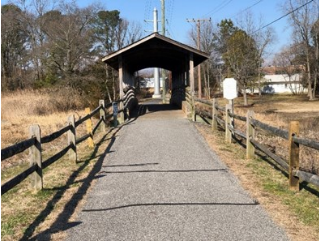
Photo 32 – St. Michaels Nature Trail Bridge over San Domingo Creek
