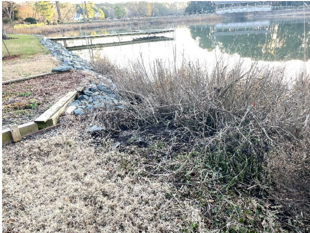
Photo 5 - Revetment and Natural Banks along Private Properties
