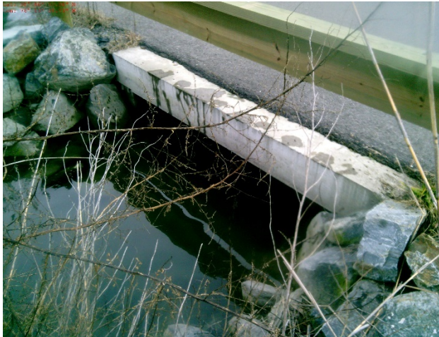
Photo 19 - Grace Street Culvert (looking SE)
