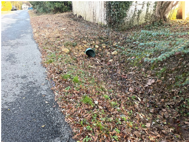
Photo 23 – Grassy Swale along Southern Road Edge
