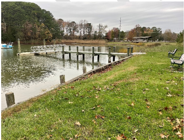
Photo 30 - Pier and Floating Dock Infrastructure
