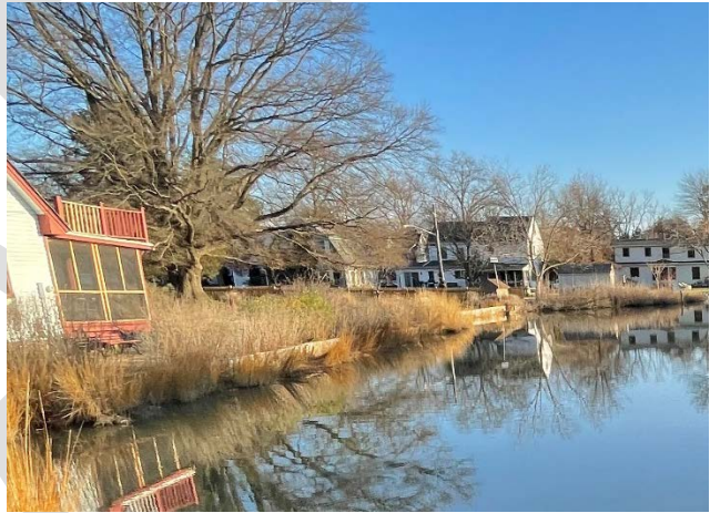
Photo 6 - Bulkhead along Private Property
