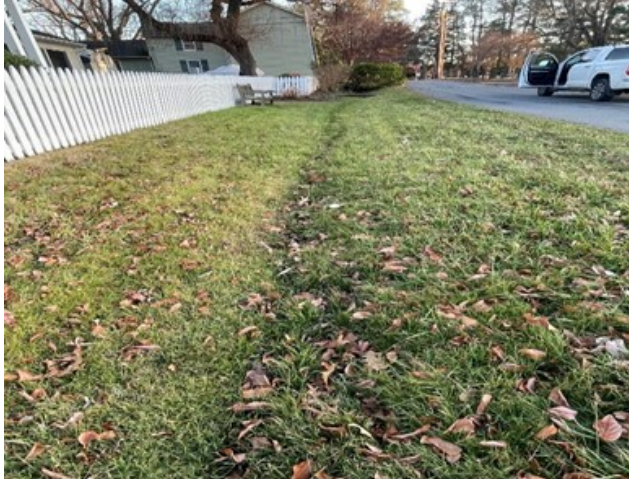
Photo 25 - Grassy Swale along Tilden Street
