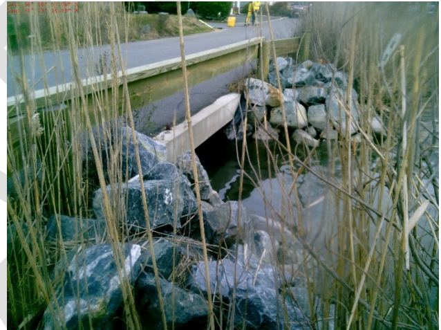
Photo 20 - Grace Street Culvert (looking NE)
