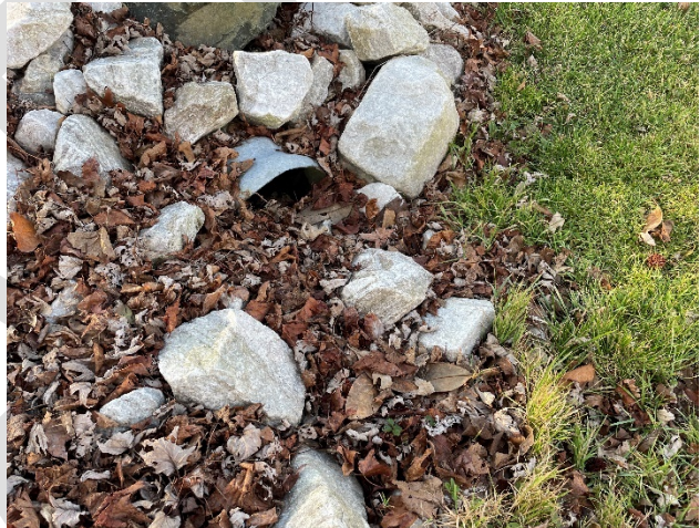
Photo 16 - Outfall along Swale at Canton St.
