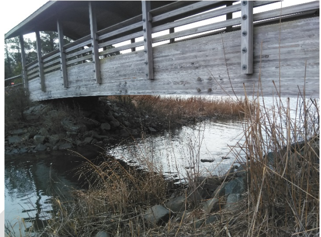
Photo 33 - Bridge Structure along Trail
