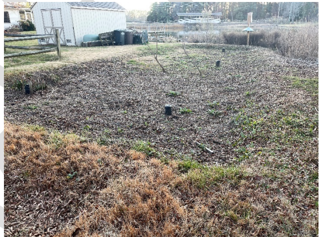
Photo 24 – Retention Pond at Thompson Street
