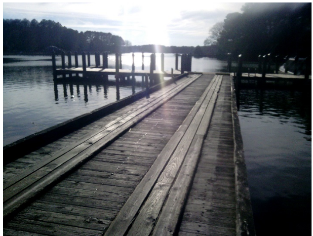
Photo 31 - Fixed Pier for Docking along San Domingo
