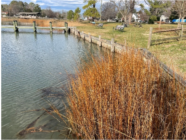
Photo 3 - Bulkhead at Back Creek Park
