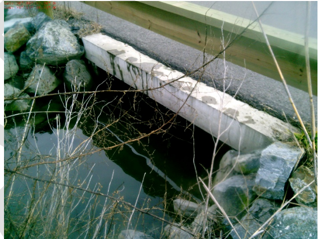
Photo 12 - Grace Street Culvert
