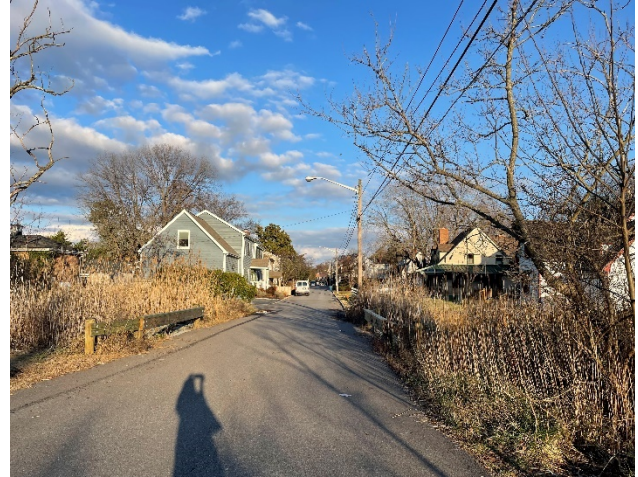
Photo 18 - Grace Street at Culvert (looking East)
