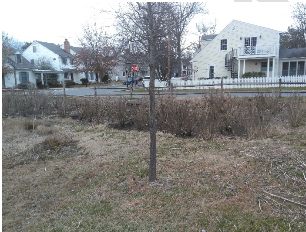
Photo 23 - Retention Pond at Intersection of W. Chestnut and Tilden Streets
