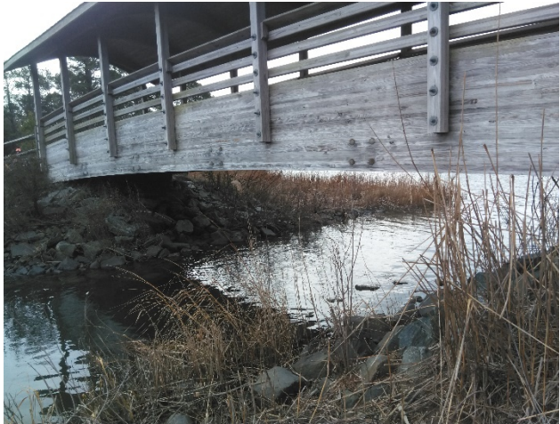
Photo 11 - St. Michaels Nature Trail Culvert
