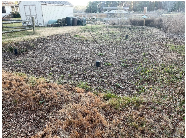
Photo 24 - Retention Pond at Thompson Street
