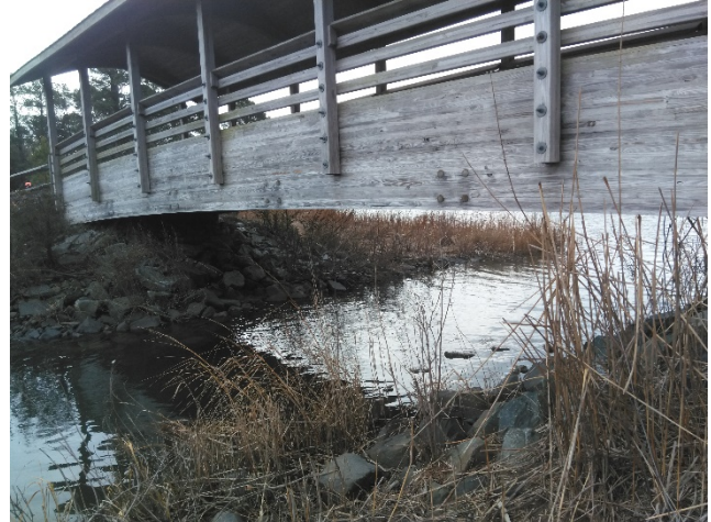
Photo 37 - Bridge Structure along Trail
