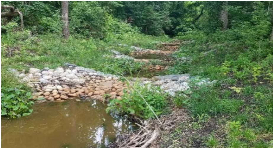
Photo 45 - Riffle-Pool Conveyance System
