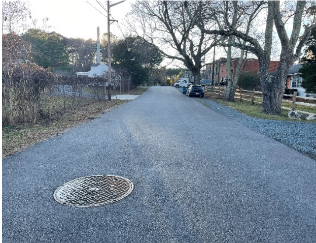
Photo 13 - Canton Street (looking West)
