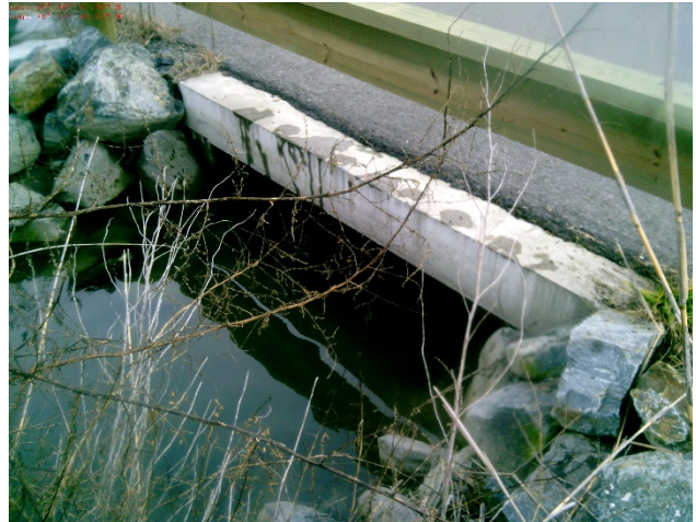
Photo 12 - Grace Street Culvert
