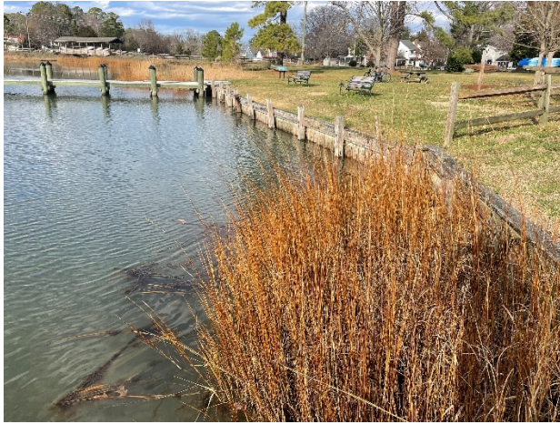
Photo 3 - Bulkhead at Back Creek Park
