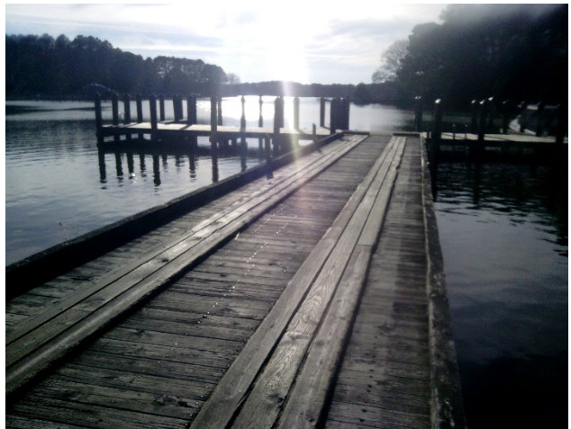
Photo 35 - Fixed Pier for Docking along San Domingo Creek
