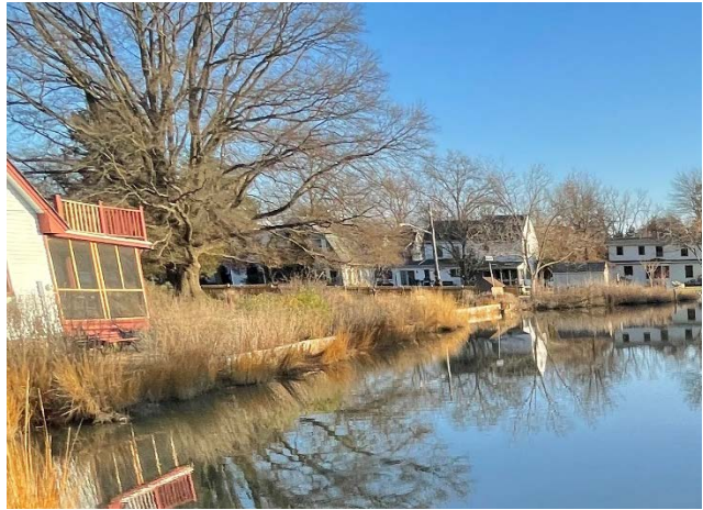
Photo 6 - Bulkhead along Private Property
