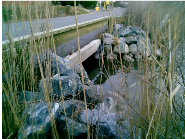
Photo 20 - Grace Street Culvert (looking NE)
