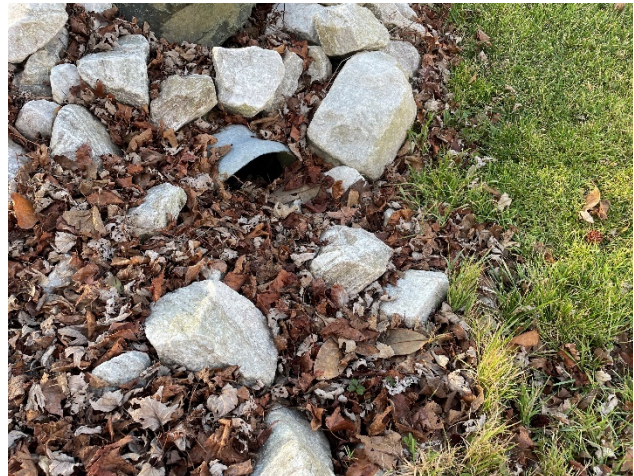
Photo 16 - Outfall along Swale at Canton St.
