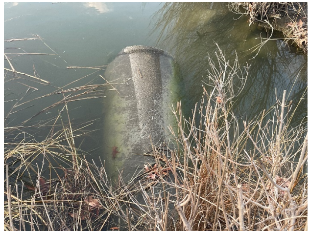
Photo 28 - Outfall Pipe from Retention Pond at W. Chestnut St. and Tilden St.
