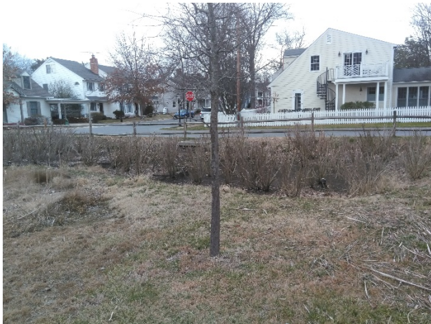
Photo 27 - Retention Pond at Intersection of W. Chestnut and Tilden Streets
