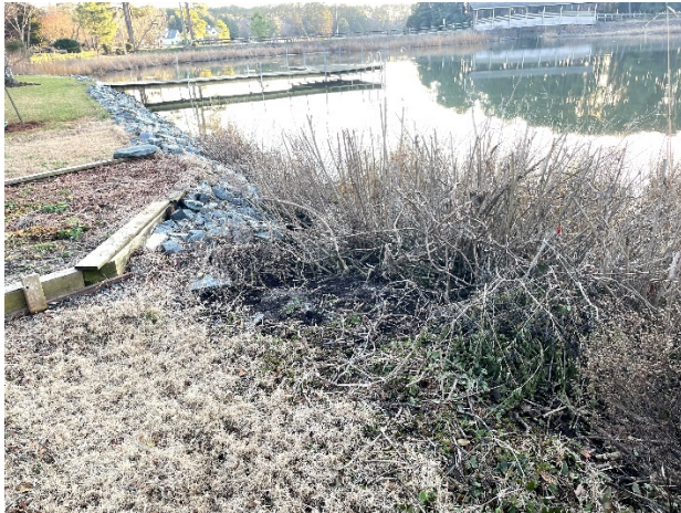
Photo 5 - Revetment and Natural Banks along Private Properties
