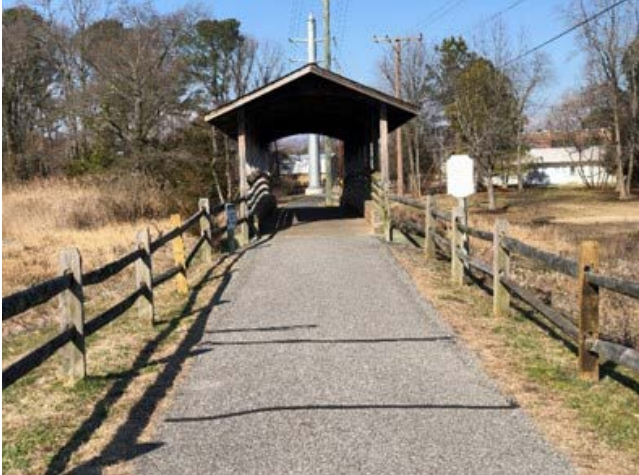
Photo 36 – St. Michaels Nature Trail Bridge over San Domingo Creek
