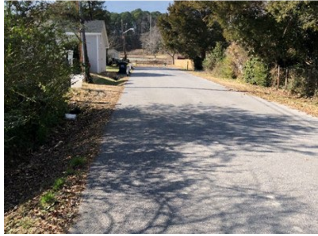
Photo 22 - Thompson Street (looking West)
