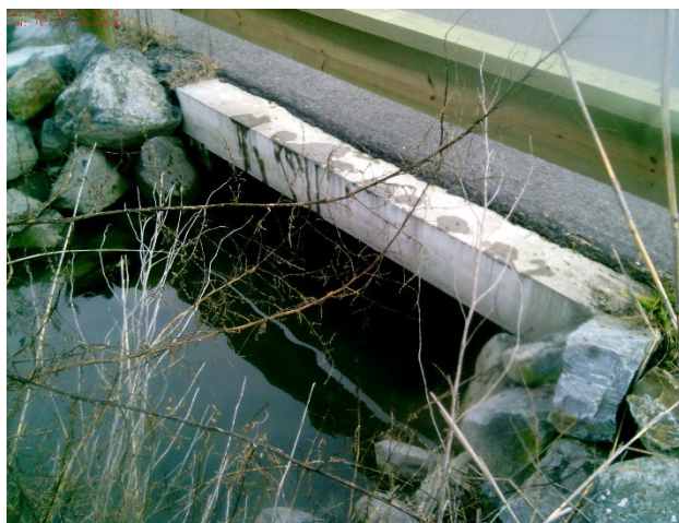
Photo 12 - Grace Street Culvert
