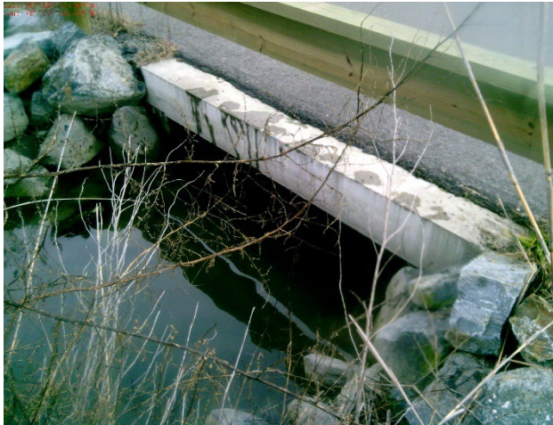
Photo 19 - Grace Street Culvert (looking SE)
