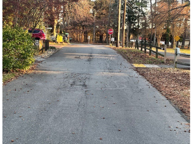
Photo 26 - Tilden St. (looking South)
