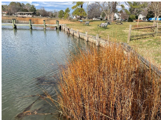
Photo 3 - Bulkhead at Back Creek Park
