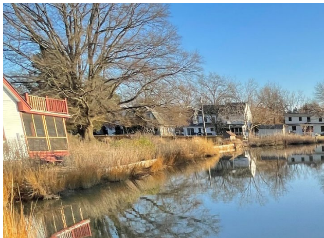
Photo 6 - Bulkhead along Private Property
