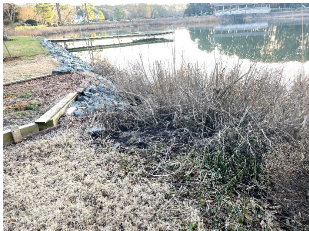
Photo 5 - Revetment and Natural Banks along Private Properties
