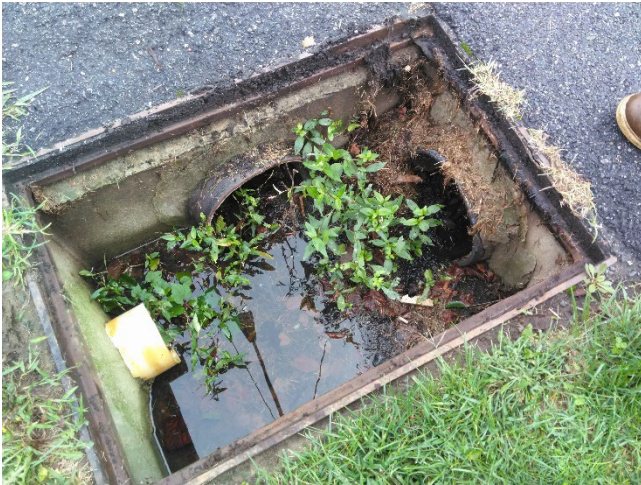
Photo 49 - Existing inlet with sedimentation
