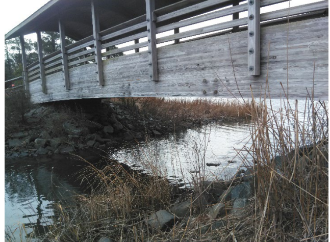
Photo 37 - Bridge Structure along Trail
