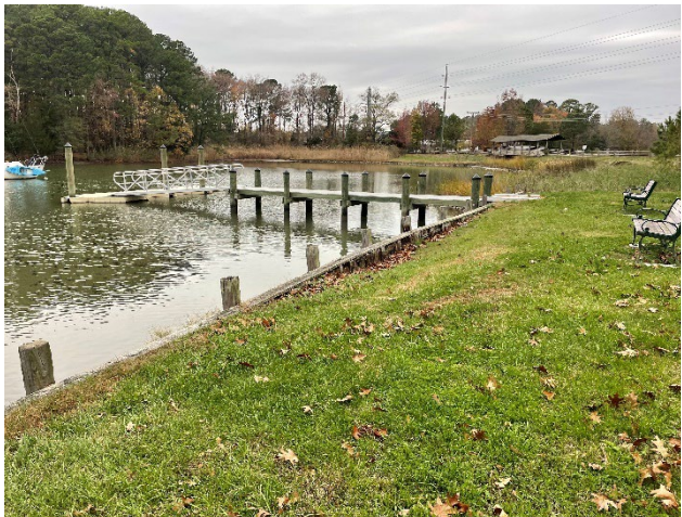
Photo 34 - Pier and Floating Dock Infrastructure
