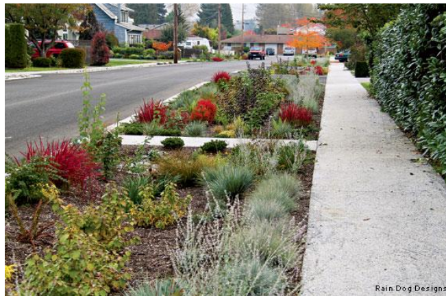
Example of a raingarden retrofit in previous parking area.
