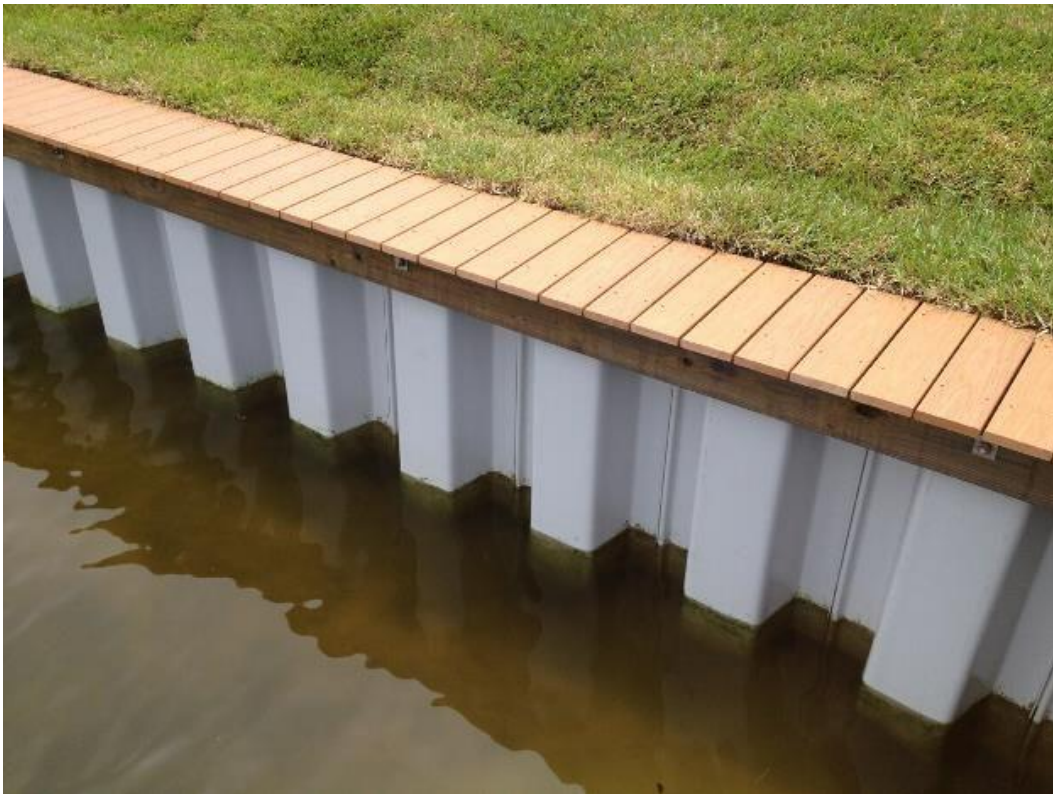
Example of a shore Guard vinyl sheet piling bulkhead with wooden top cap. The top cap can be expanded to encompass the boardwalk.
