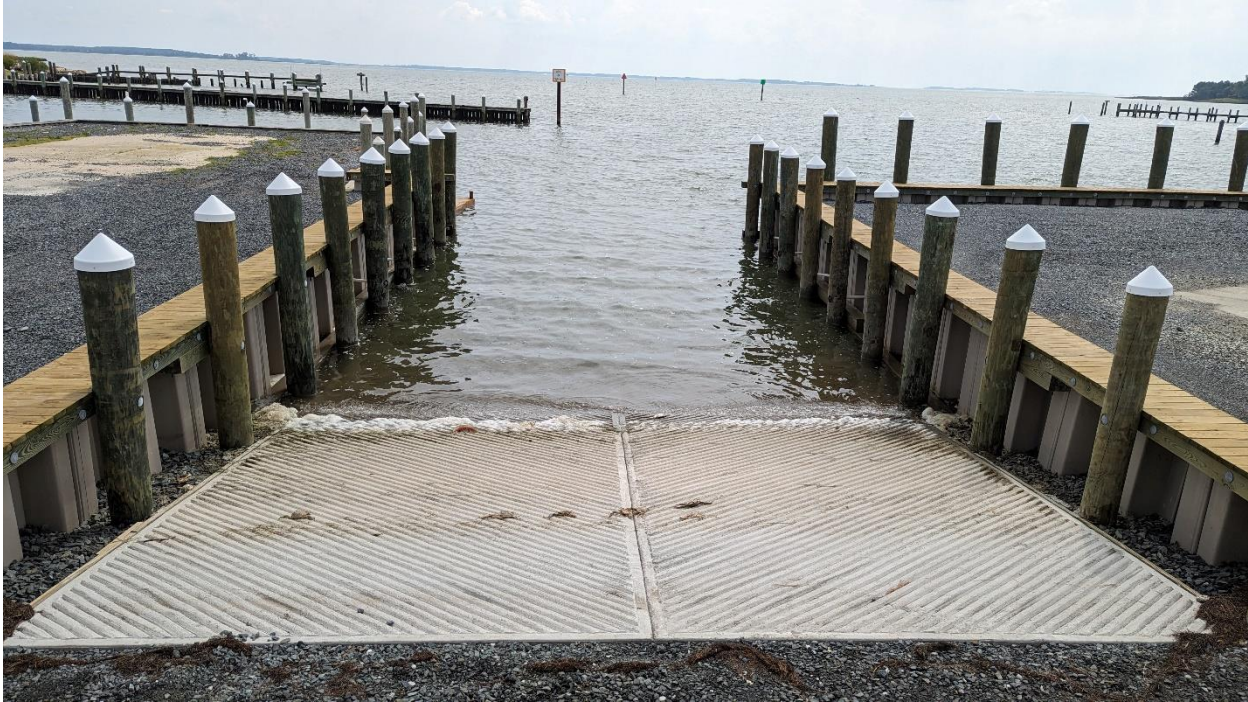
Example of a newly completed boat ramp designed by GMB
